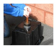
Mark a circle in the centre of the bottom of the box, a little larger than the diameter of the cutter. This is purely a guide to allow the hole to be cut centrally.
